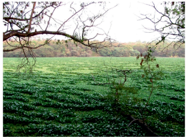
Present condition of Katraj lower reservoir
